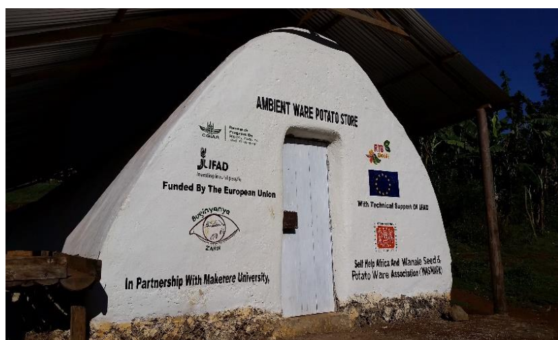
Fig. 1. Ambient storage structure
